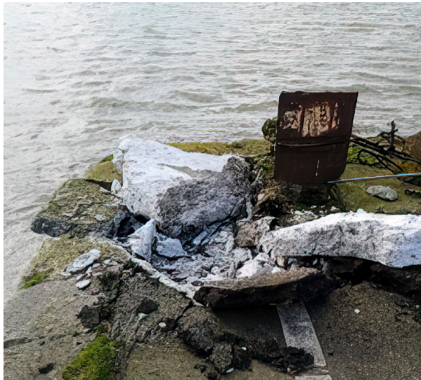
Bollard ripped from the quay. (Source: Wagenborg)
