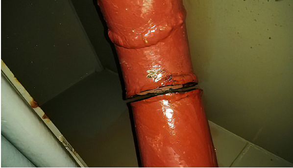
Broken fire extinguisher pipe Zealand Delilah. (Source: Q-Shipping)
